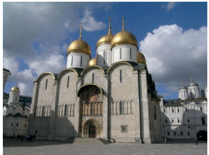
Photograph of the Cathedral of the Dormition today (Figure 1)
